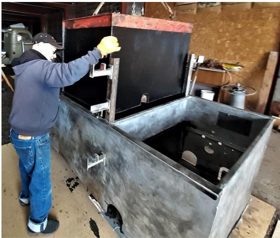
Mike Johnson oversees installation of the water tank.
