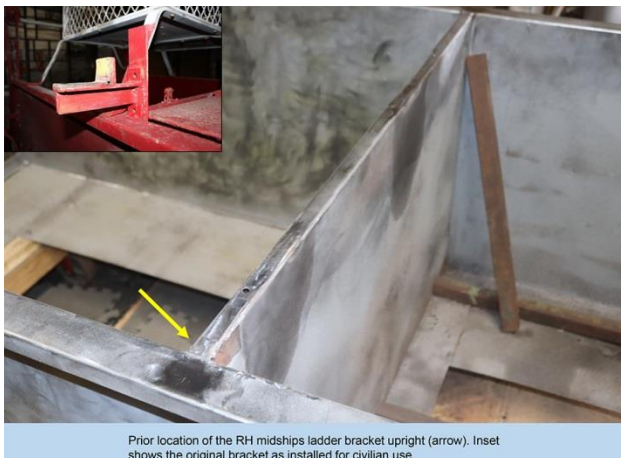
Rust repairs inside of tank bay.
