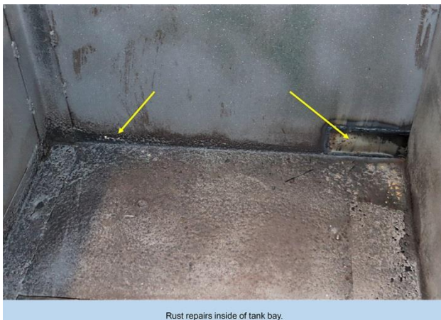
Rust repairs inside of tank bay.
